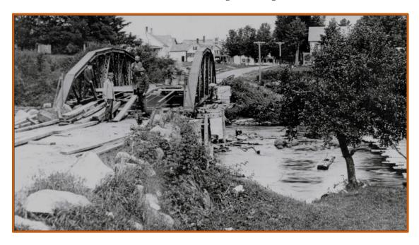
This view toward Freedom shows a crew installing the wooden deck on the Effingham span. During the construction period, pedestrians utilized a temporary crossing made of planks lashed together and laid atop rocks in the river, downstream from the new bridge (visible at the far right).
